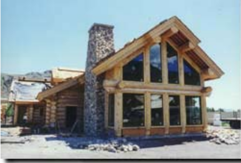
A scribe fit log home - courtesy of A Place In The Sun Log Homes, Inc. North America).
