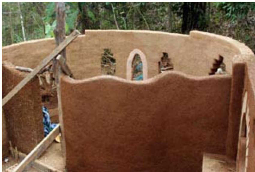
Cob house construction (source: http://www.sgnb.com/ )
